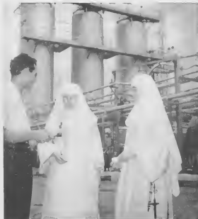
Against a background formed by the No. 2 Alky Plant, a Lago tour leader shows two Sisters samples of oil processed by the unit.
